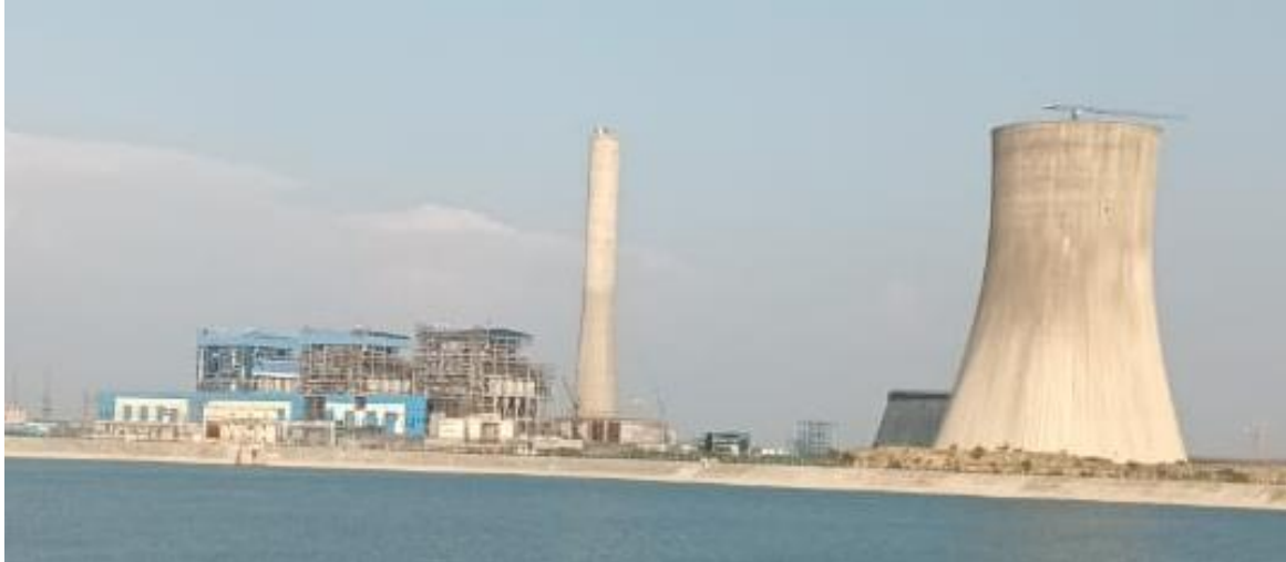
View of Ghatumpur Thermal Power Plant
